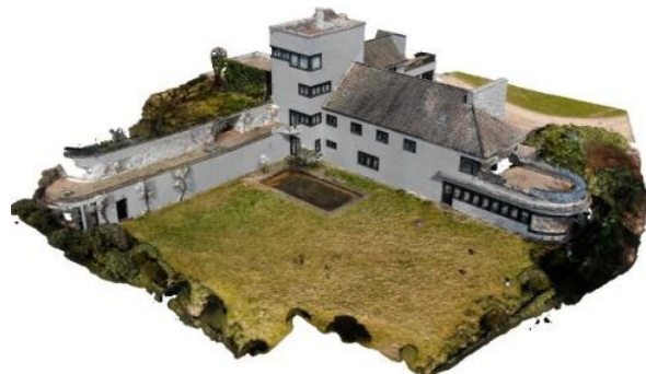
Figure 5. Coloured point cloud from terrestrial and UAV photogrammetry.
