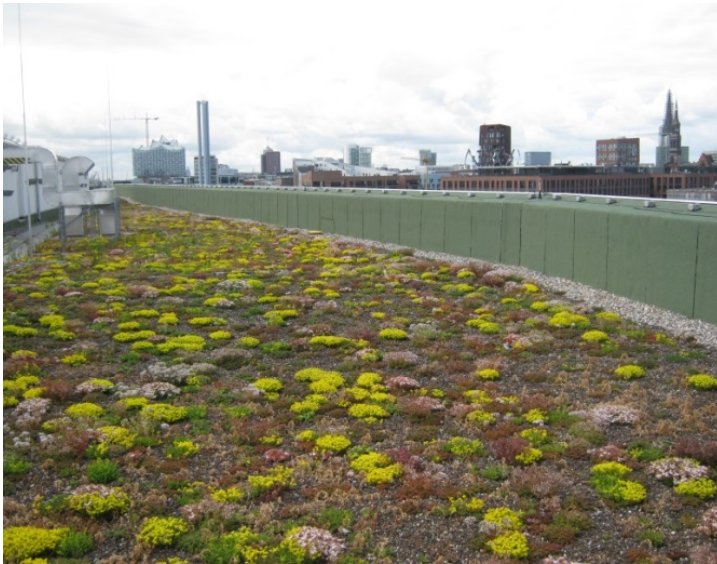
Fig. 2 View over the HCU green roof
