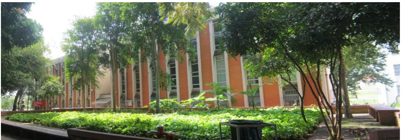
Fig. 2: Southwest view of the campus building IFCH Campinas
