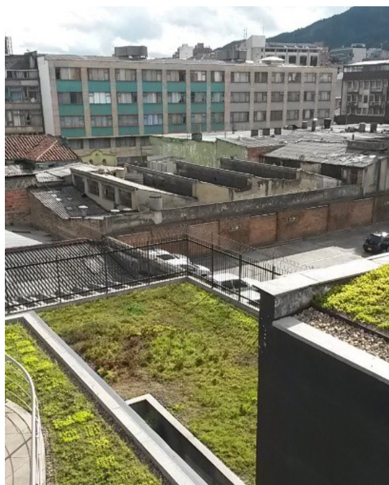
Green Roof and Vertical Garden systems installed on the Bogota Secretary of Environment following initial WSUD policy
