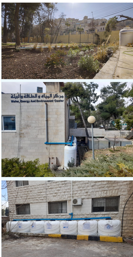
Figure 17: Water Harvesting Systems Installation Source: (UN Habitat and GAM 2023)
