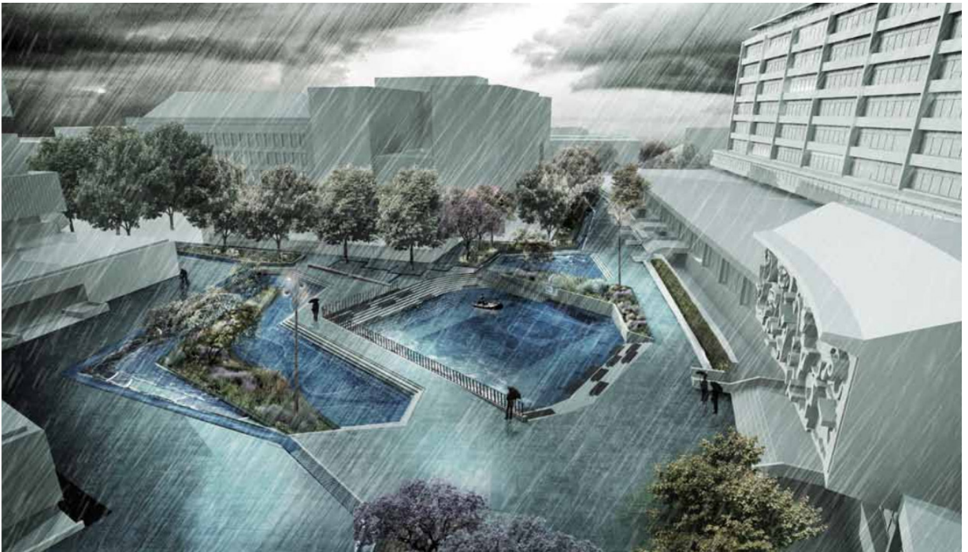
Figure 20: The Bentheplein water square as temporary water storage facility, artist's impression of the scene during a downpour (top) ; The Bentheplein after a shower (bottom left) and on a sunny day (bottom right) Source: (Rotterdam Climate Initiative 2013)
