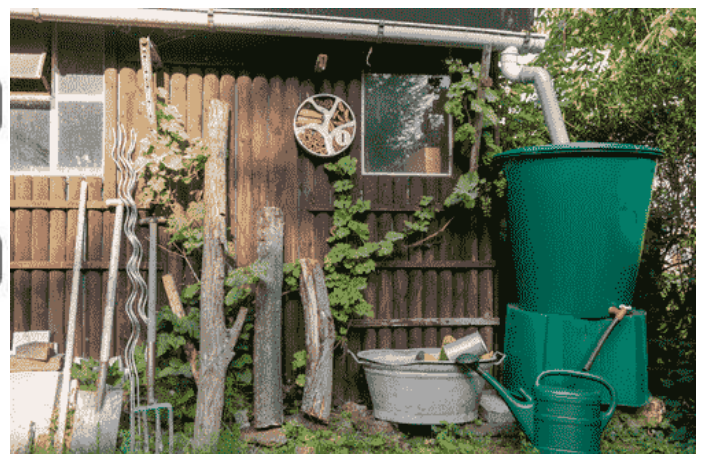
Figure 29: RWH in a garden for irrigation Source:(UltraTech Cement 2021)
