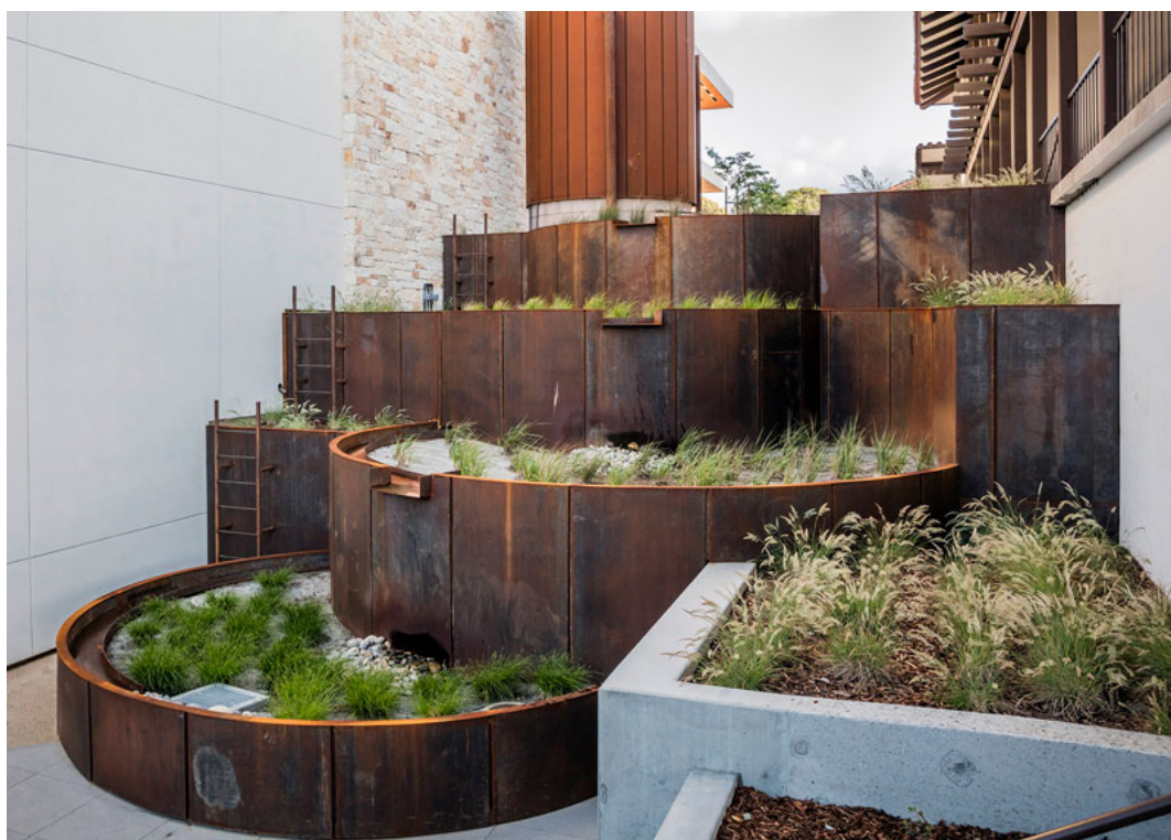
Figure 27: A series of stormwater planters collecting water between two structures integrated into the landscape, creating a drainage chain to reduce runoff volumes and rates, Source: (Central Steel Service Inc 2019)
