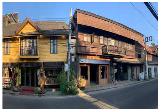
Figure 2: The lower floor of these buildings in the Wat Ket community is used for commercial purposes, while the upper floor of the buildings is for residential use. The building on the far-right side of the photo also shows how materials are often mixed with concrete or cement being used for the lower floor while the upper floor remains wooden (Photography: School of Public Policy, CMU, December 2019)
