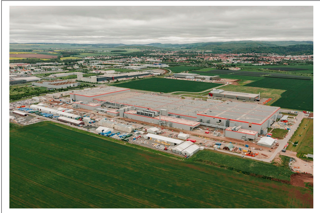
Figure 3. Construction site of CATL's EV battery cell gigafactory at the Erfurter Kreuz industrial park in Arnstadt-Ichtershausen, Thuringia; Image: Marcus Glahn, 2024.
