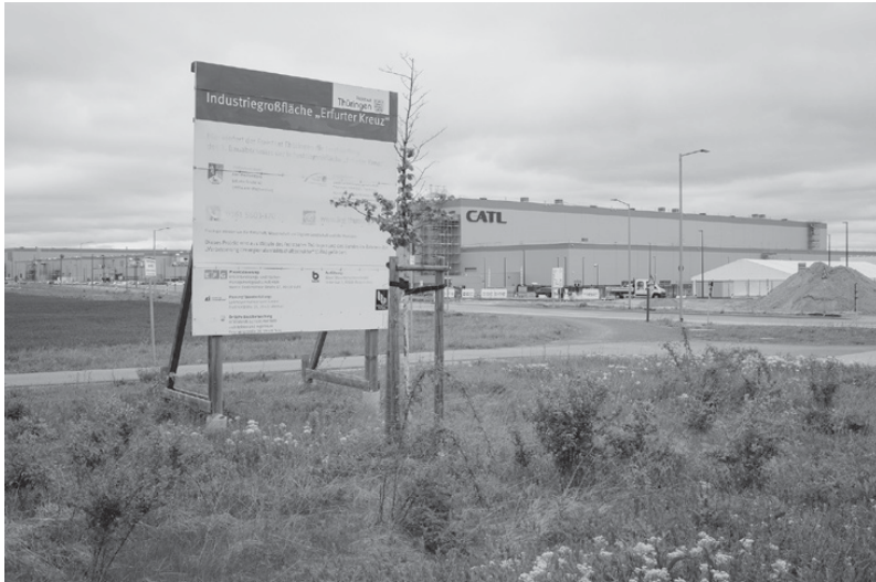
Figure 5.1: Construction noticeboard for Erfurter-Kreuz industrial site in Arnstadt-Ichtershausen. In the background is the construction site of the new gigafactory for manufacturing electric vehicle battery cells by the Chinese corporation CATL.
