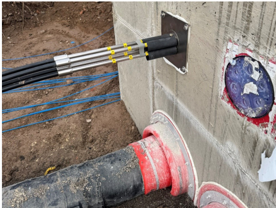
Figure 8: Rod-Extensometer applied to Shaft-Wall
