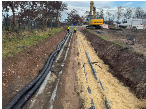
Figure 7: Backfill with different Materials for test-fields
