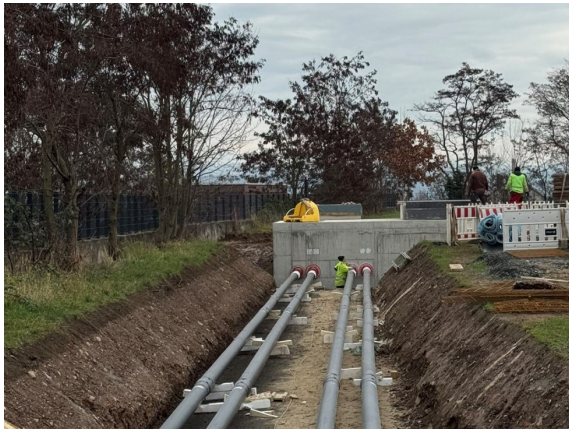
Figure 6: Trenching with sloped Walls
