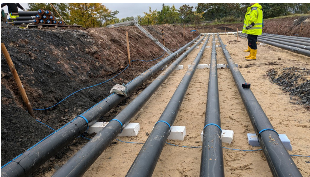
Figure 9: Installation of the fibre-optic measuring cable on the pipes by winding it around them and on the slope using wooden pegs.
