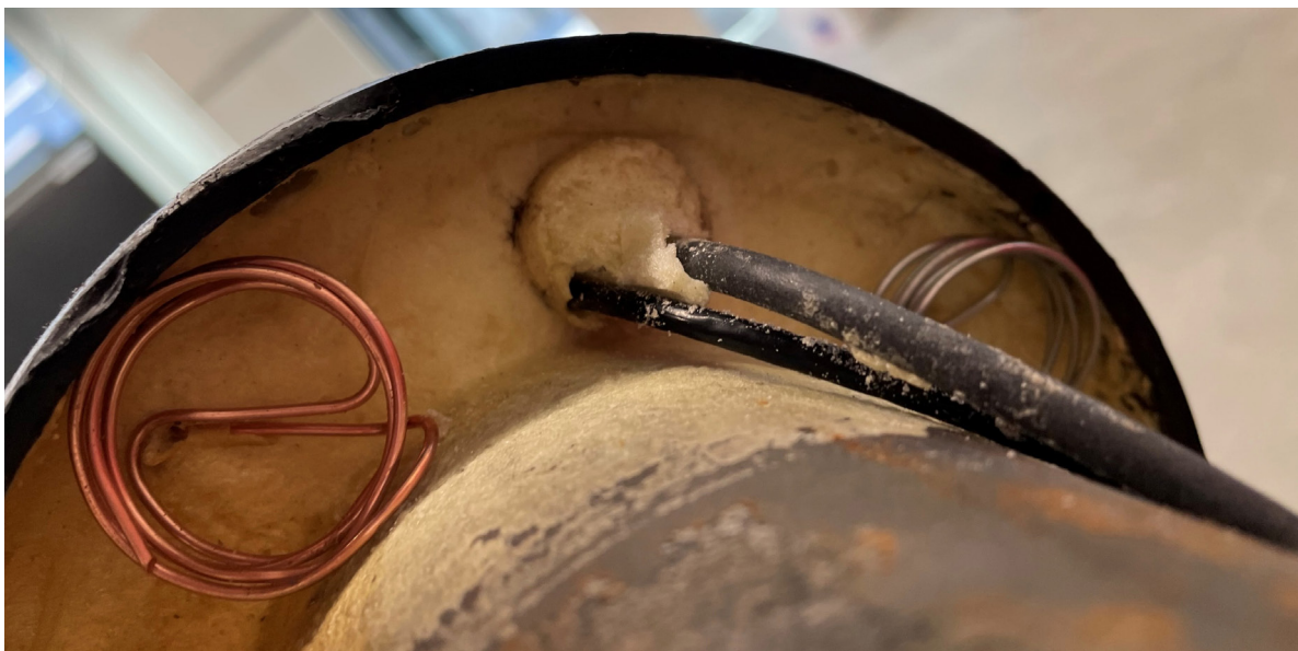
Figure 13: Sensors foamed into the pipe
