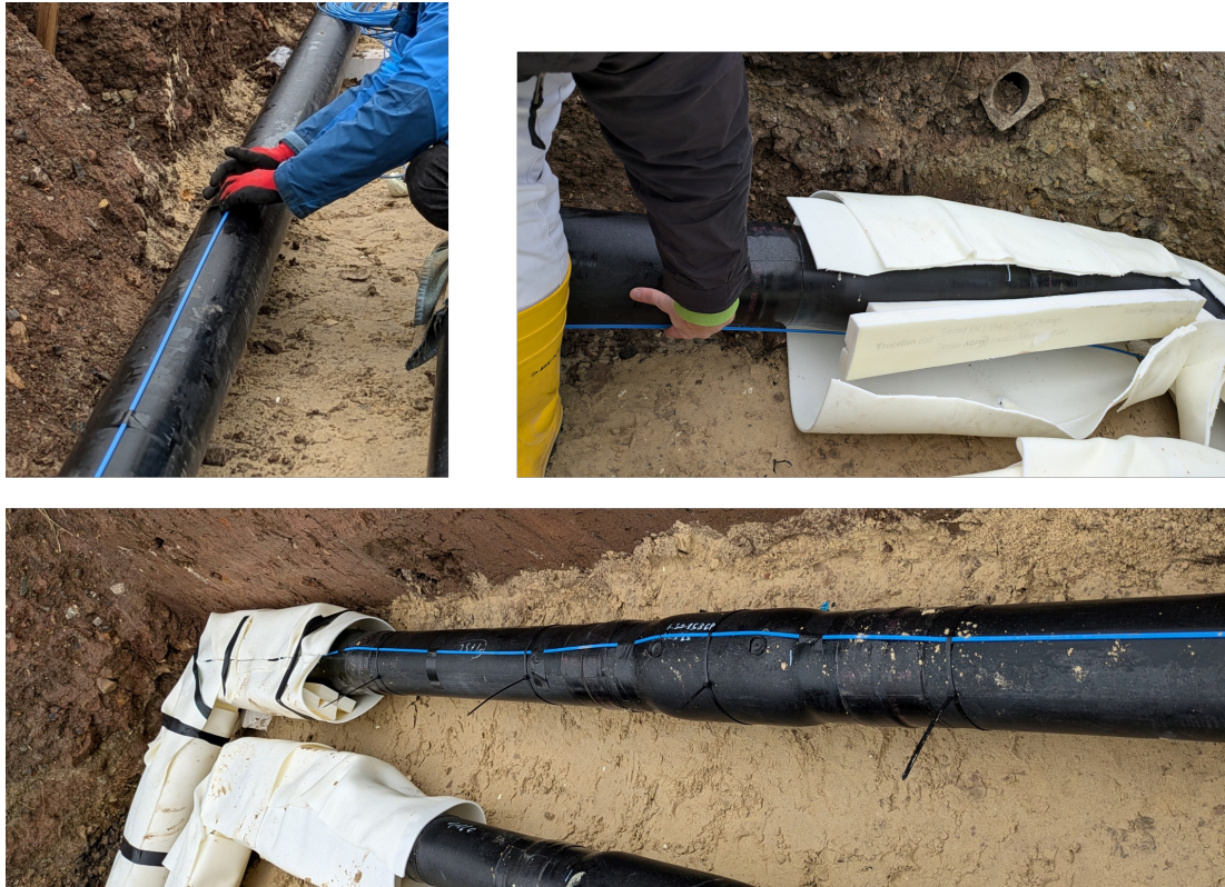
Figure 6: Installation of the fibre optic cable on the outer pipes
