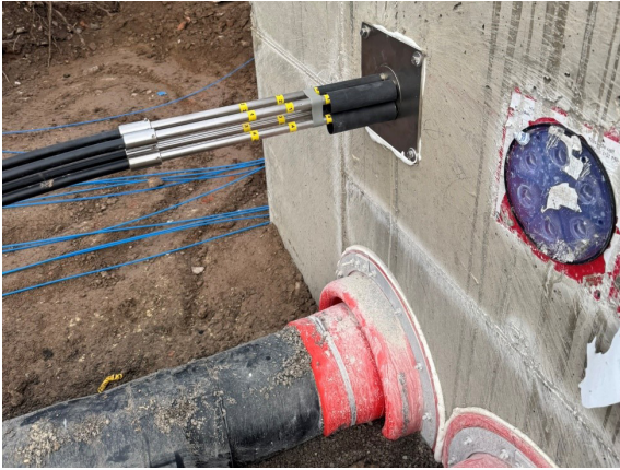
Figure 8: Rod-Extensometer applied to Shaft-Wall
