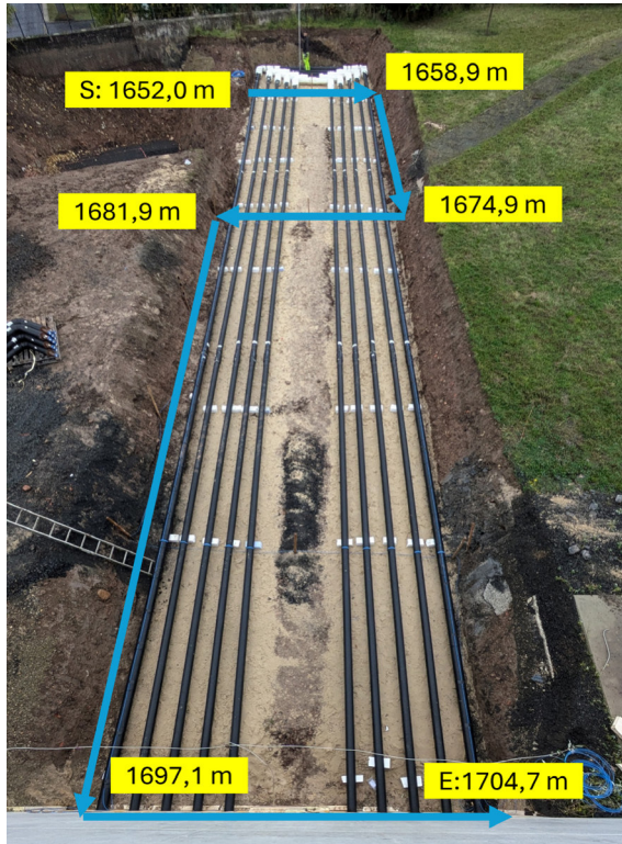
Figure 10: Cable routing on the level between the pipes
