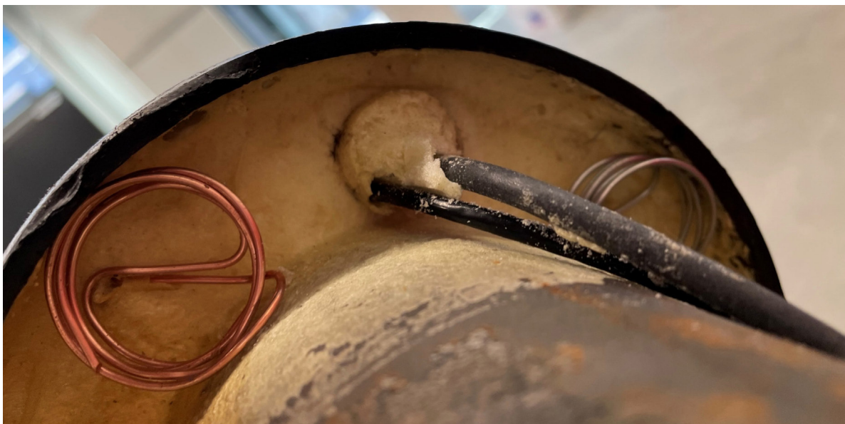
Figure 13: Sensors foamed into the pipe
