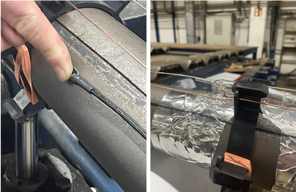
Figure 12: Installation of the humidity and temperature sensor and the surface temperature sensor in the pipe
