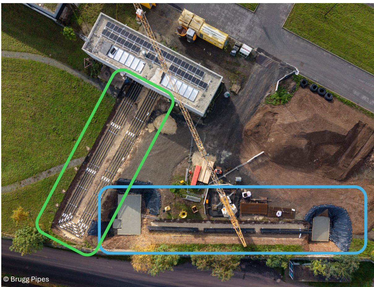
Figure 4: Aerial view of the District LAB during construction work, with the experimental fields “pipe test bench” (blue) and “flexible heating grid” (green) marked.
