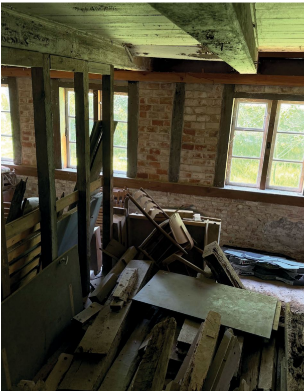
Fig. 2.3.5: Photo of obstacles in the Hufnerhaus
