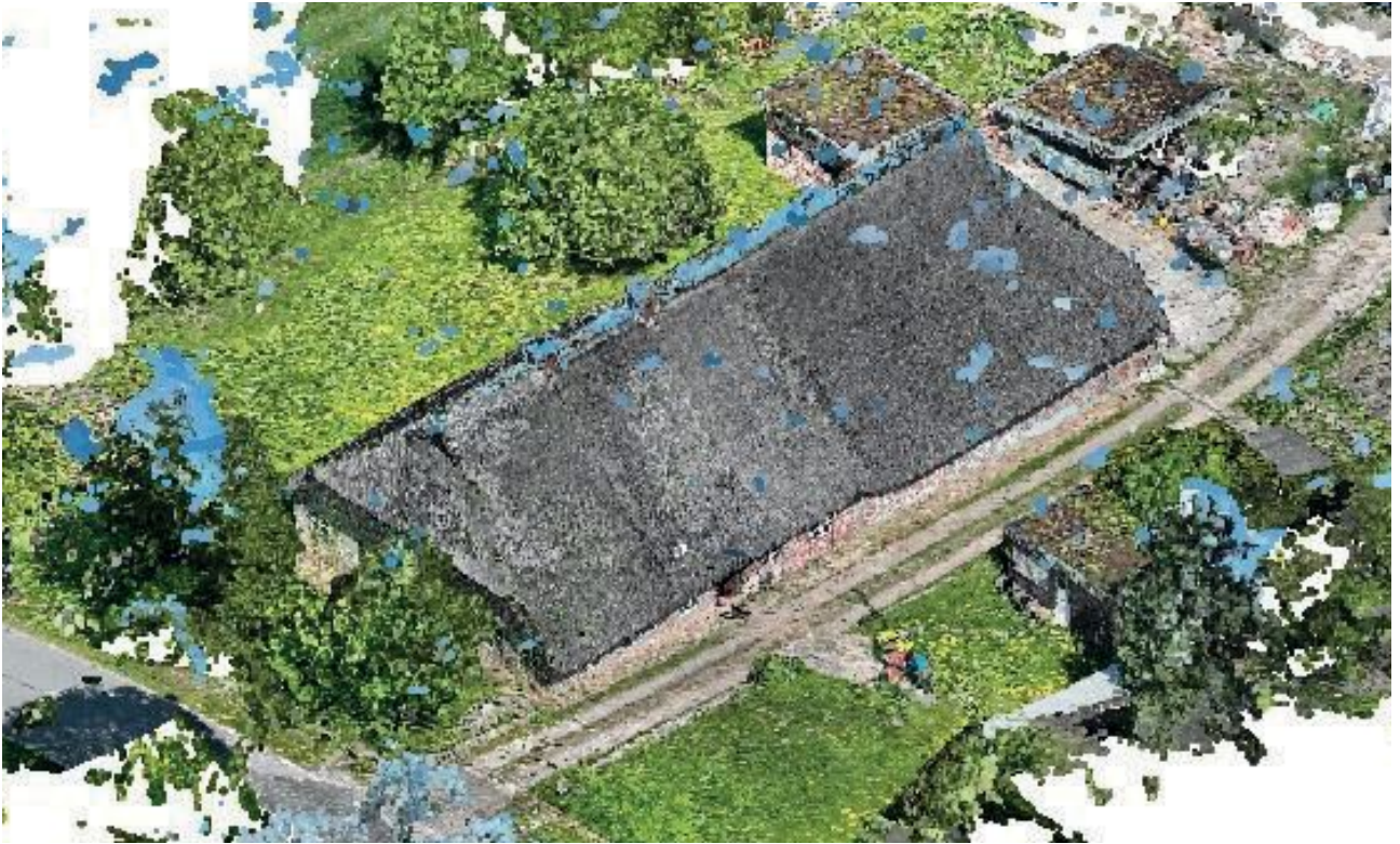
Fig. 1.4.6: 3D point cloud from WebODM in Archicad
