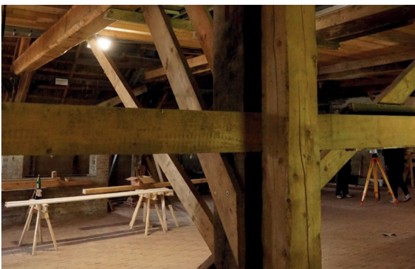
Fig. 4.3.7: photos around column
