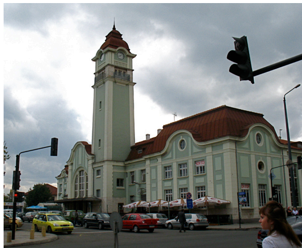
Fig.14: Main train station, nowadays / http://en.wikipedia.org/wiki/File:Burgas_Central_Railway_Station_Mihal_Orela.jpg
