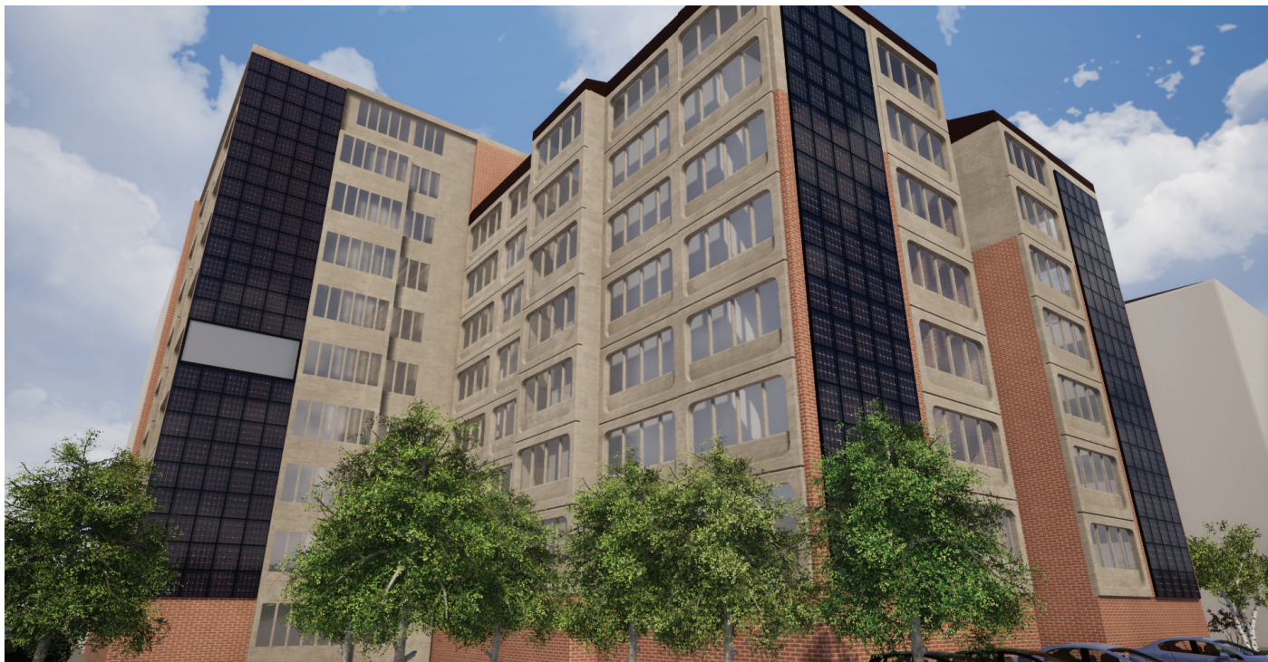
FIGURE 42 - Intervention proposal through Insulation and photovoltaics.
