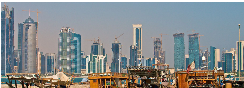
Fig.1.1 | Doha skyline under construction
