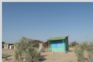
Fig 7.2.2 Bassisa's street side shop
