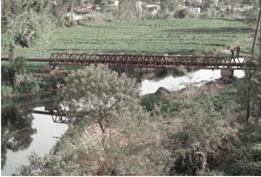
Fig. 6.1.11 water supply pipe as pedestrian bridge, Mekanissa (source: photo by author)
