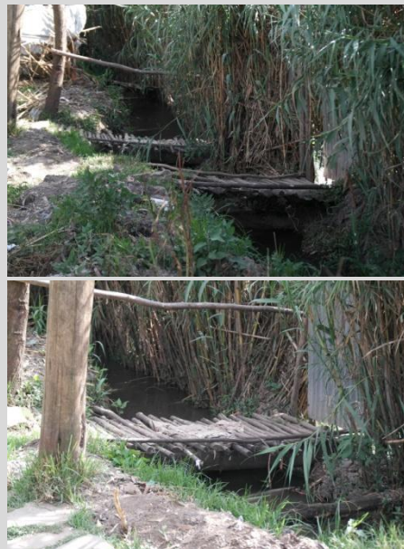
Fig. 6.1.14 'Shenbeko' filtration and guiding channel wall
