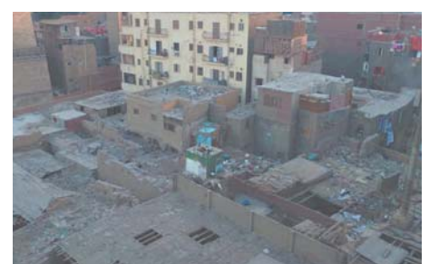
Fig. 3: Roof tops in El Gamaleya
