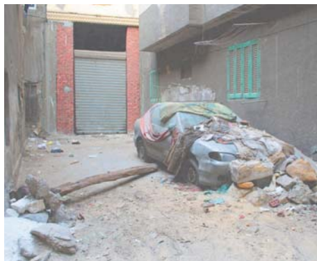
Fig. 2 Degraded buildings in El-Gamaleya
