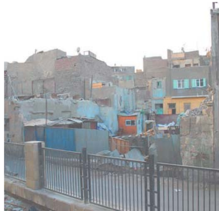
Fig. 4 Degraded buildings in El-Gamaleya
