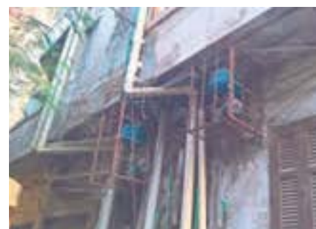
Fig. 5: Typical infrastructure for water supply and wastewater seen in El Gamaleya
