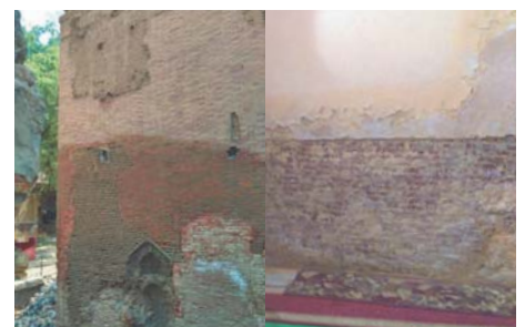
Fig. 4: Damage caused to buildings by rising groundwater levels
