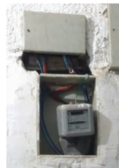
Figure 14: Energy consumption tracking meter at a resident's house in Sheikh Zayed, Cairo. (Rayaprolu, 2017).
