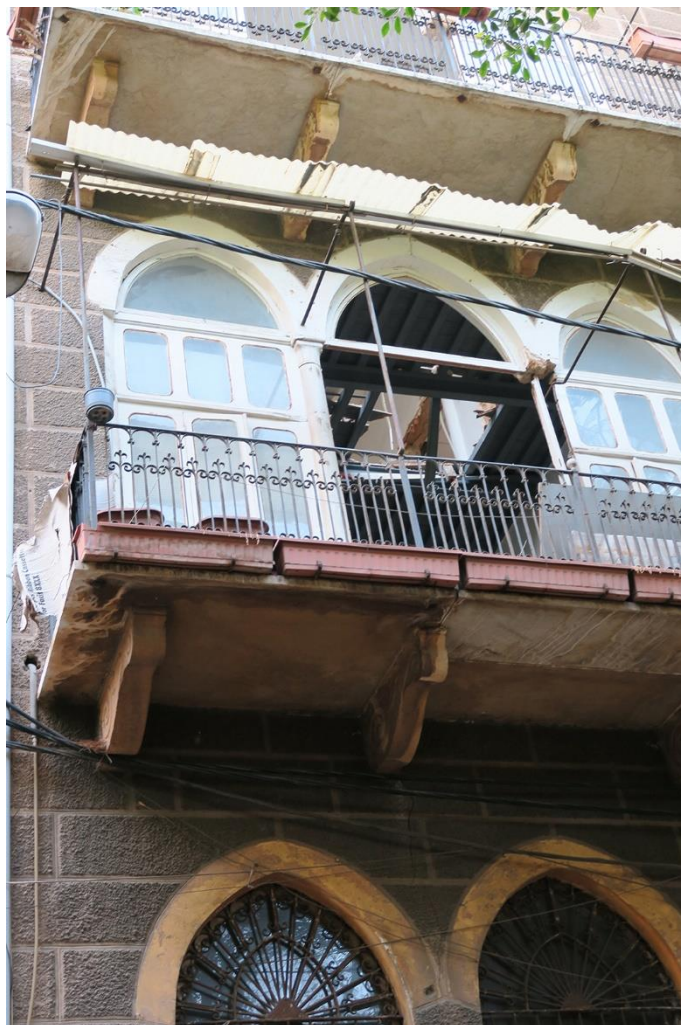
Image 16: An early twentieth century building on Ibrine Street in Furn al-Hayek, which was intentionally left to decay. Photo by author, 2017.
