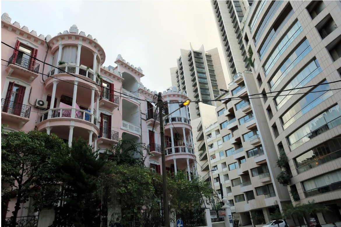
Image 11: Balconies in Furn al-Hayek Street according to the previous (to the left) and to the current Construction Law (to the right). Abdel Wahab 618 towers are seen in the background.
