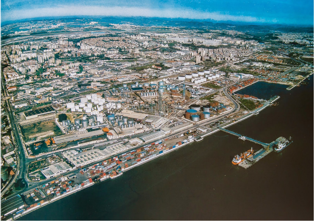
Figure 47. Expo location before the construction start. We can see several industries, including a petrochemical area that was later transferred to Sines. Retrieved from www.skycrapercity.com
