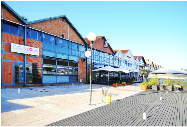
Figure 50. Refurbished warehouses for restaurants and bars in Doca de Sto. Amaro. This project preceded the POZOR, but already indicated the transformation path of disuse port areas for leisure activities. Project from architect Rui Alexandre. Photo: José M Pagés Sánchez
