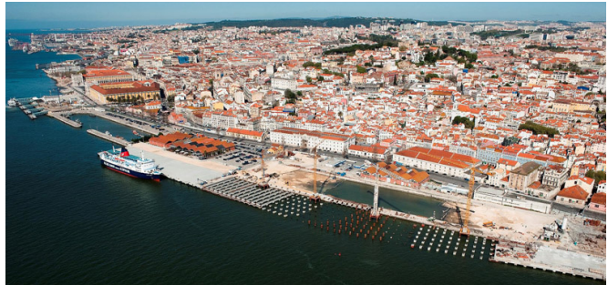
Figure 74. View of the area where the cruise terminal was built, during the construction period of the dock. Source: https://tpf.eu/wp-content/uploads/2007/01/Jardim-do-Tabaco-Quai-Lisbonne-800-400.jpg
