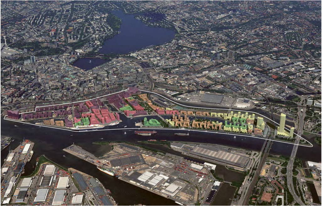
Figure 29. General view of the Hafencity project. The western section is almost completed, while the eastern it is starting to be built. Source: Hafencity GmbH
