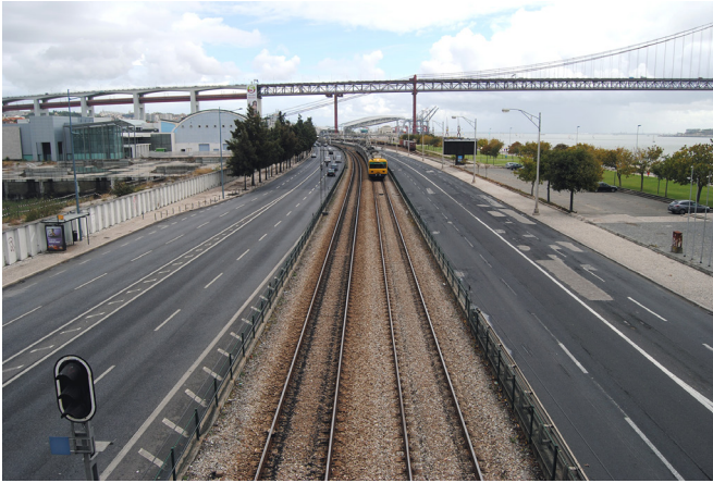
Figure 54. Roads and railway line form a barrier separating the city from the river, also in the areas where there are no port activities. Despite several attempts since the 1970s, the issue has not been solved. In other cases, explored in Ch. 4, we saw that one of the first actions to redevelop the waterfront was burying the road or railway (e.g. Oslo or Marseille). This solution has been proposed several times in Lisbon, but never executed. Author: José M P Sánchez
