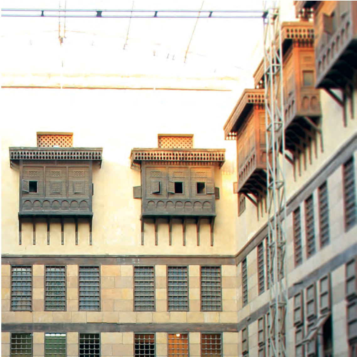
Figure VIS.4 – Traditional building – Passive systems for intercepting solar gains and mashrabiya . (Photo G. Vignola)
