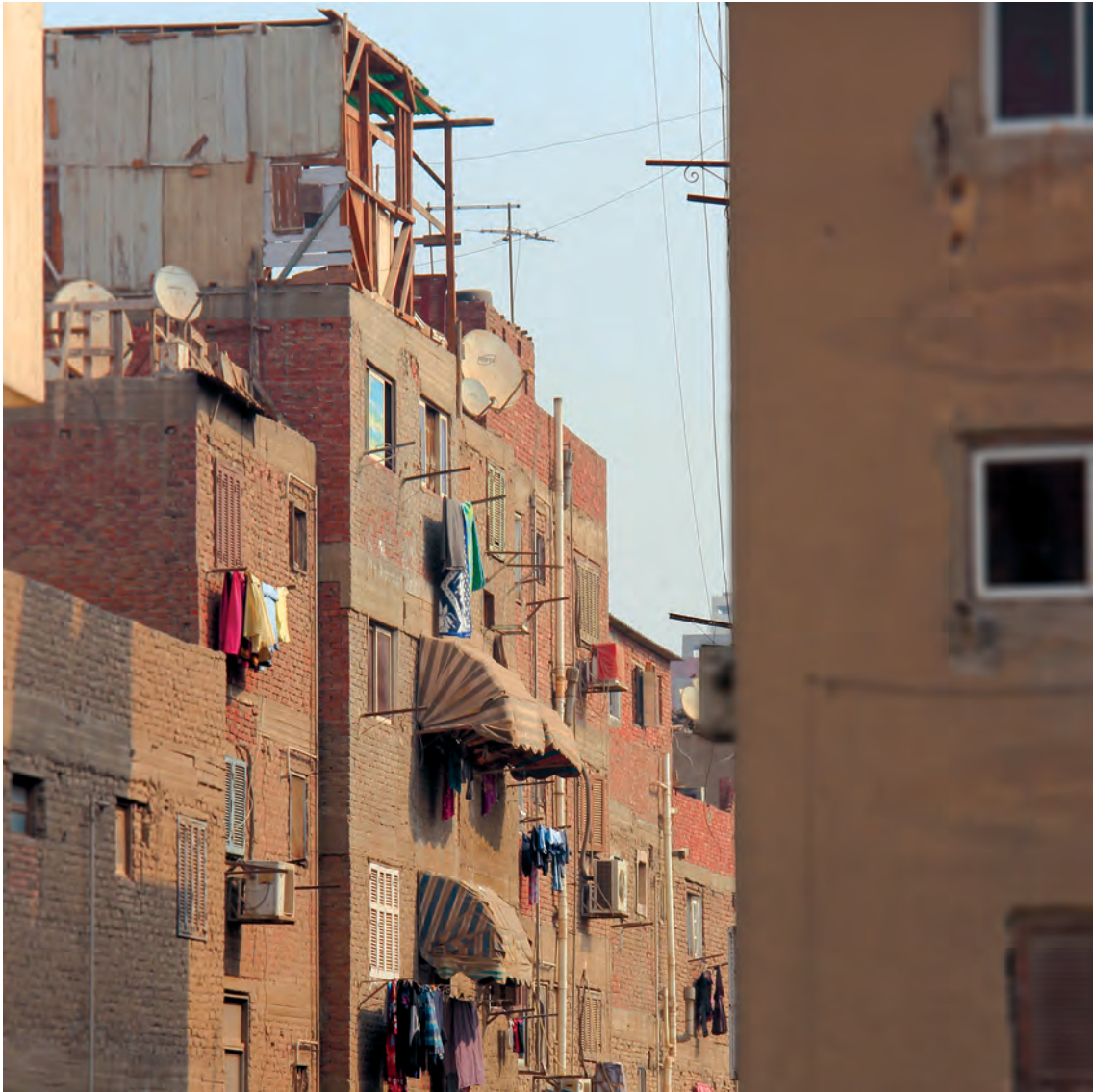
Figure VIS.3 – Informal housing – Passive systems for intercepting solar gains. (Photo G. Vignola)
