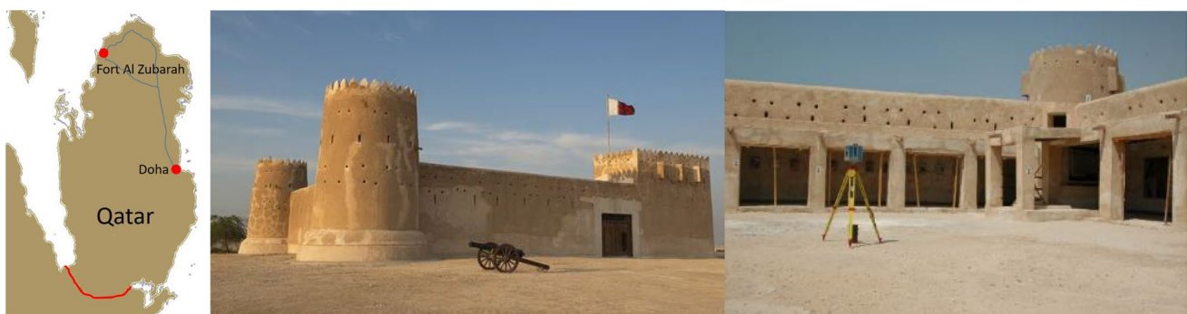
Fig. 1 The Arabic fortress Al Zubarah in Qatar—the location in the map (left), the exterior (centre) and interior with the terrestrial laser scanner (right)
