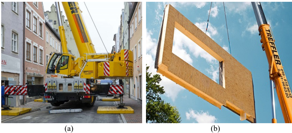
Figure 2: (a) Mobile crane; and (b) Prefabricated panel installation.
