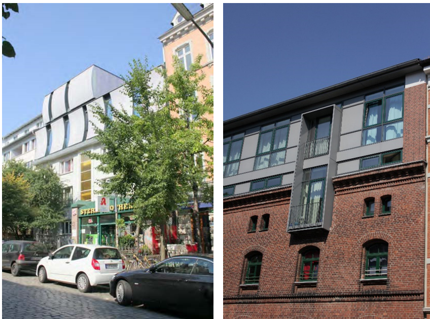
Figure 3: Examples of completed rooftop additions.
