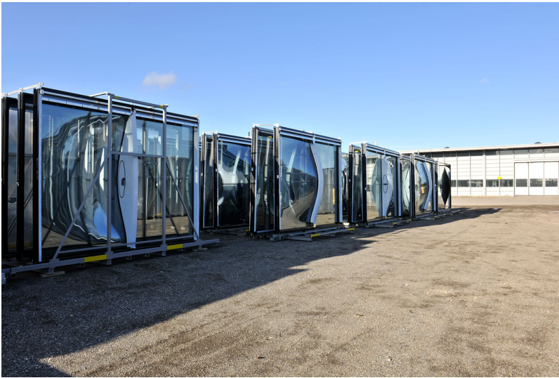
Figure 1. The innovative glass panels for the curved façade of the Elbe Philharmonic Hall, which required, among other things, the development of new glass specifications. © Stephan Liebl.
