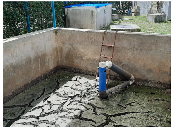
Figure 08 Faecal sludge in an unplanted drying bed (source: BORDA, 2021)
