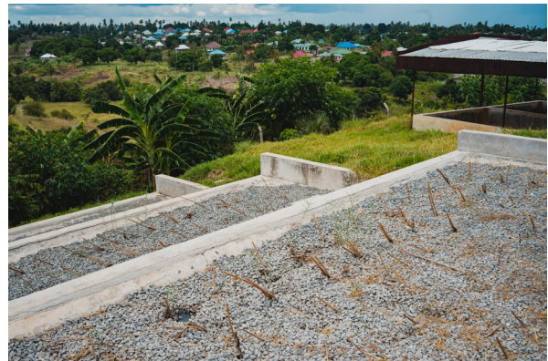
Figure 61 Planted Gravel Filters (PGF) (source: Author, 2021)
