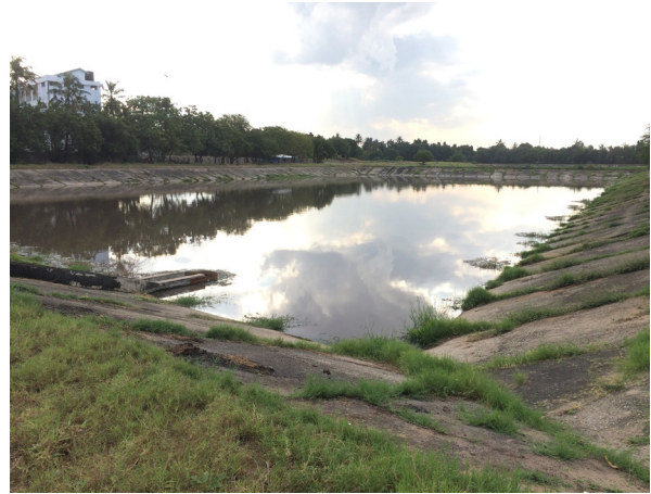
Figure 17 Waste Stabilisation Pond (WSP) in Dar es Salaam (source: BORDA, 2021)
