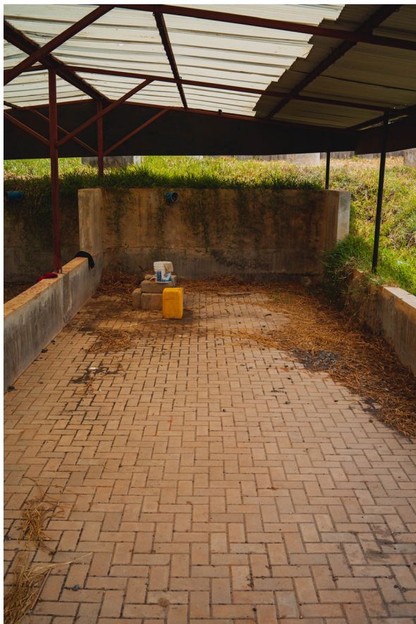
Figure 59 Sludge drying beds (source: Author, 2021)
