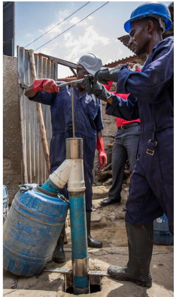
Figure 13 Service with the Gulper technology (source: BORDA, 2021)
