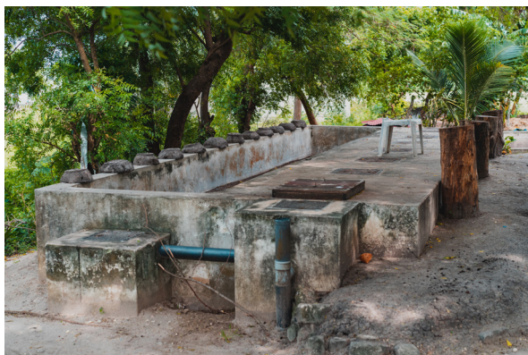
Figure 49 Unplanted sludge drying bed and drying FS soil conditioner (source: Author, 2021)
