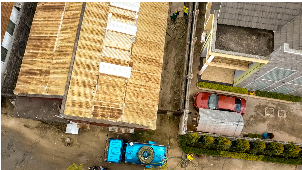
Figure 11 Vacuum truck servicing a septic tank (source: BORDA, 2021)
