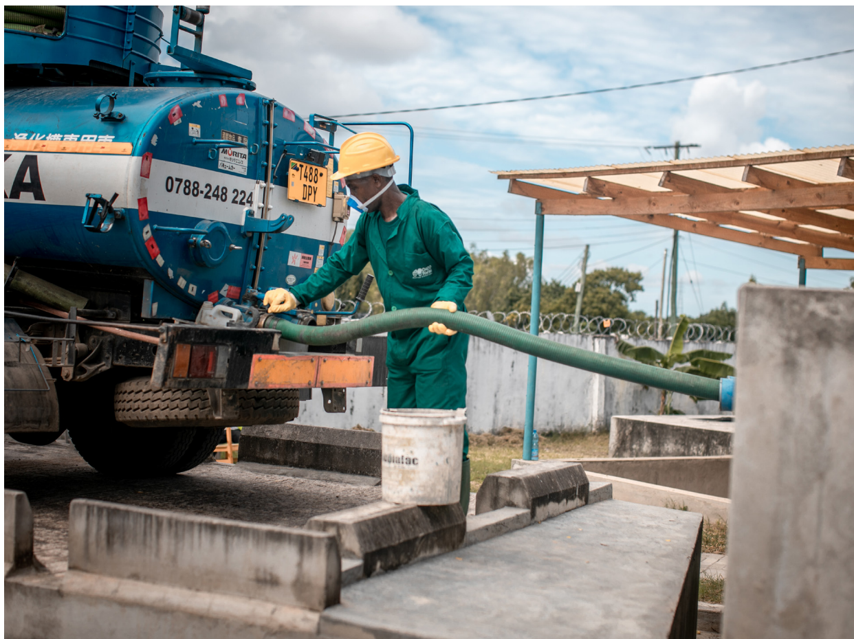
Figure 15 Emptying a vacuum truck at a DEWATS FSTP (source: BORDA, 2021)
