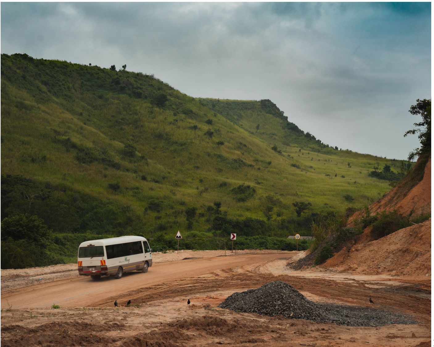
Construction of a new standard gauge rail line through Pugu Hills (Young, 2021)
