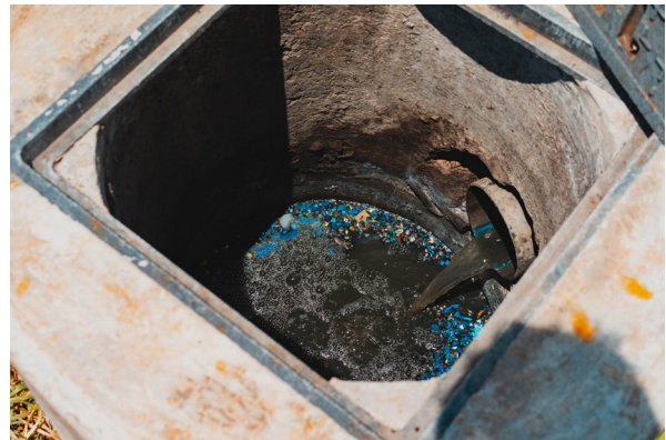
Figure 60 Expansion chamber with plastic waste (source: Author, 2021)
