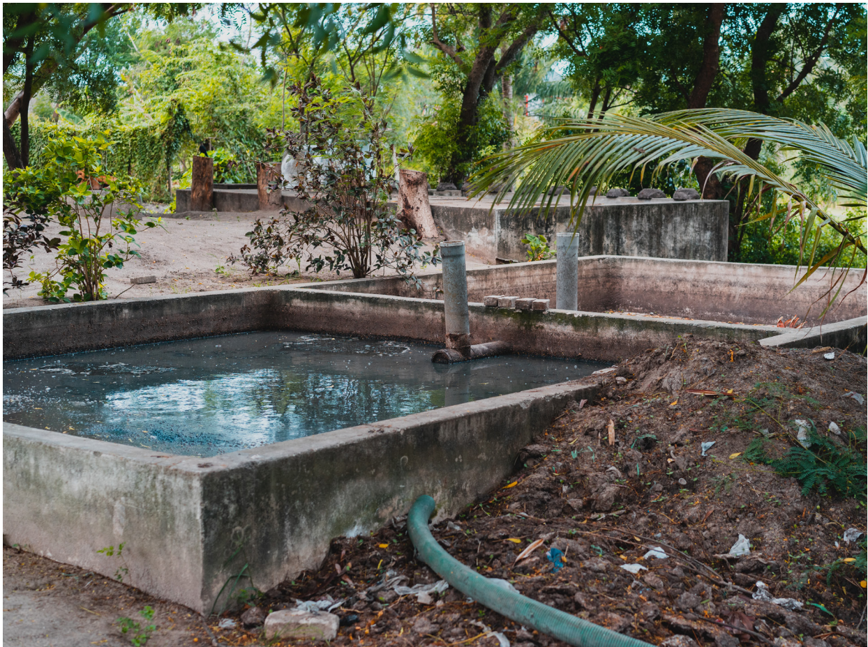
Figure 18 Unplanted drying bed at Kigamboni FSTP (source: Author, 2021)
