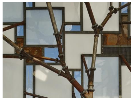
Figure 2. View of the façade from the inside
