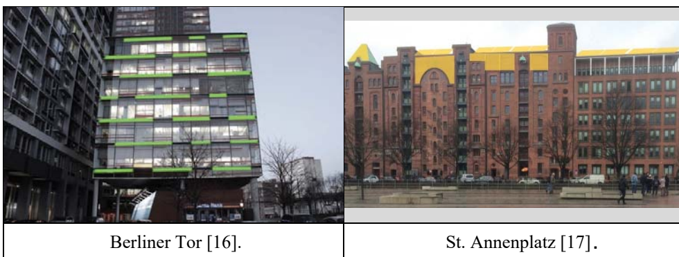
Figure 5: Proposals for the installation of PV modules in existing sunlit façades. Modules are visible from the ground level by pedestrians to improve the interest and identity of the urban space.
