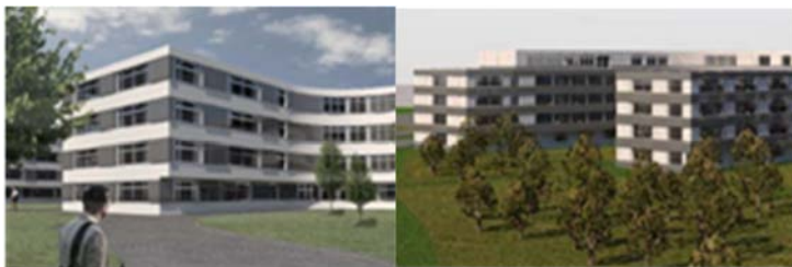
Figure 11: PV modules integrated in façades and design [9]. Left version was chosen.
