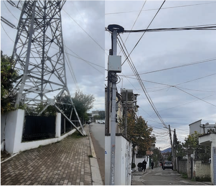
Figure 14 An Electric Pylon on a Walkway (left) and Electrical Pole (right)
