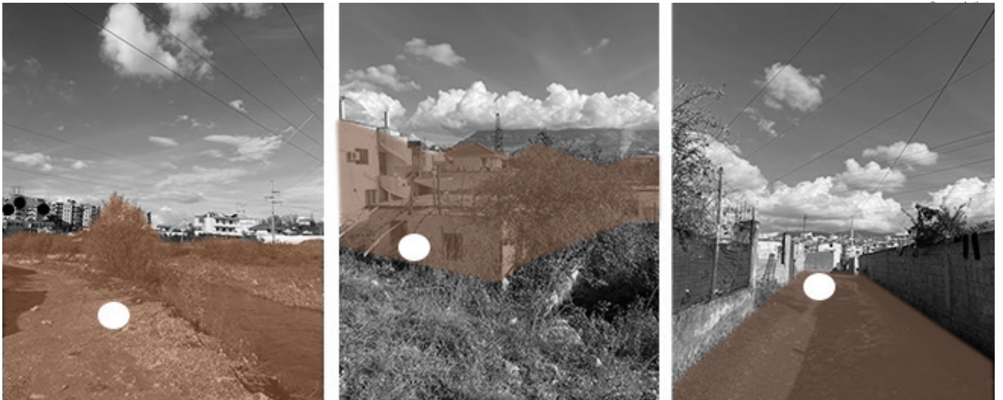
Figure 65 The Tirana River and Urban Infrastructure
