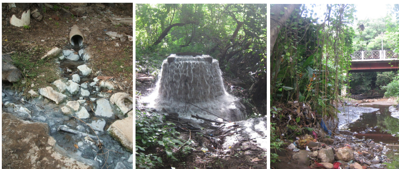
Figure 8. (From the left) A tannery's pipe discharging on the river. A blocked manhole on the riverbank. Solid waste accumulated on the river's edge (Own images, 2014)
