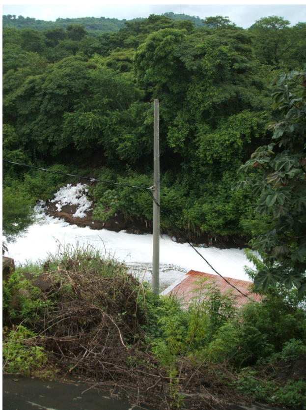
Figure 6. Discharge from Sutiava wastewater plant into Chiquito River (Own image)
