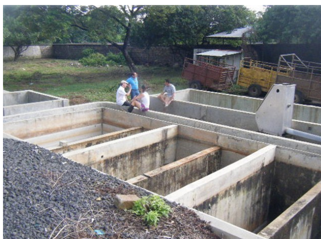
Figure 12. Infrastructure of the previous DEWATS in the slaughterhouse (BORDA, 2013)
