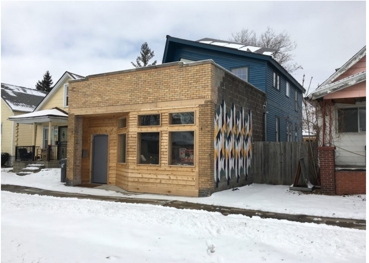
Figure 5.13: Popp's Emporium in Winter. Courtesy of Popp's Packing.
