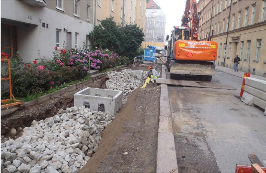
Figure 2:30 Planting beds utilizing recycled concrete instead of granite stones (Embren, 2013).
