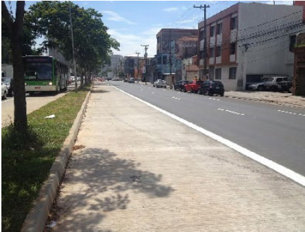
Figure 2:12 Bus corridor at Av. Rio Branco (SPTrans, 2013).
