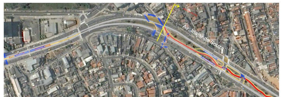
Figure 2:15 Typical Section, segment of Av. Inajar de Souza Bus Rapid Transit system in São Paulo (SPObras, 2014).
