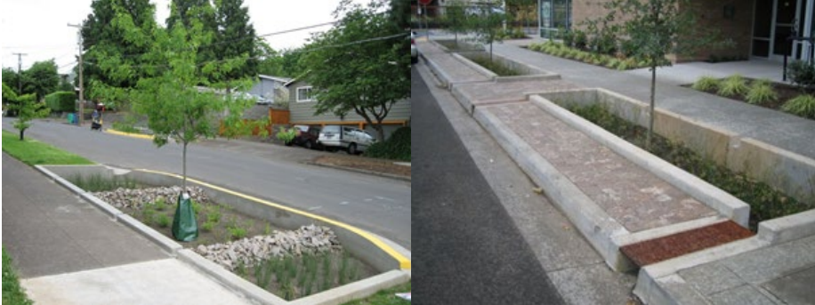
Figure 2:32 Stormwater planter design in the streets of Portland, Oregon, USA (City of Portland, 2014).
