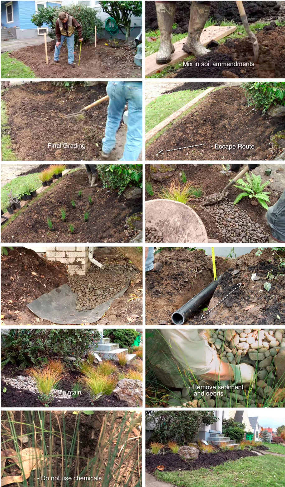
Figure 2:35 Still images of step-by-step video “How to Build a Raingarden” (City of Portland, 2012).
