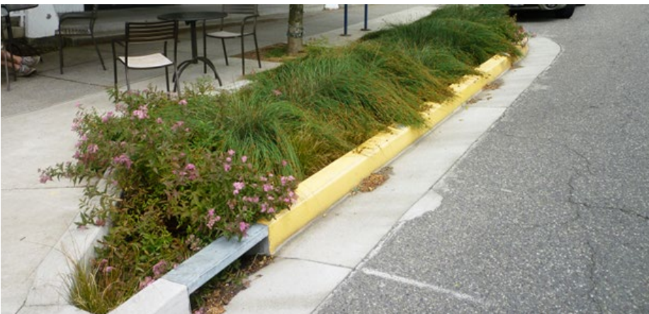
Figure 2:33 Stormwater planter with inlet from Capitol Highway and 34th Street in Portland, Oregon (City of Portland, 2014).
